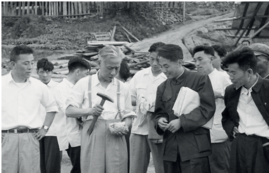
In May, 1960, Chairman Liu Shaoqi was at Sandouping, inspecting the geological structure of the dam site of Three Gorges Project.
