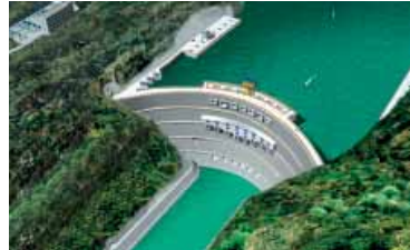
Xiluodu Hydropower Plant (under construction)
