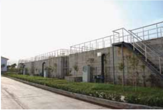
Xiangjiaba Domestic Sewage Treatment Plant
