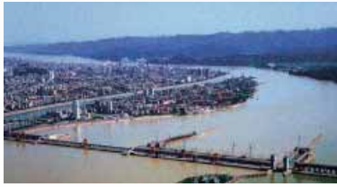
Gezhouba Hydropower Plant (completed)
