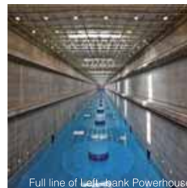
Full line of Left-bank Powerhouse
