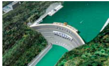
Xiluodu Hydropower Plant (under construction)
